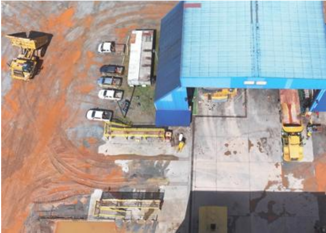
Existing condition of the maintenance wash bay 2
