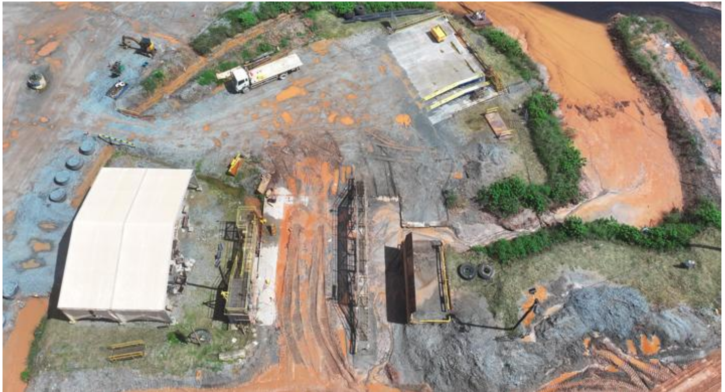
Existing condition of the maintenance wash bay 1
