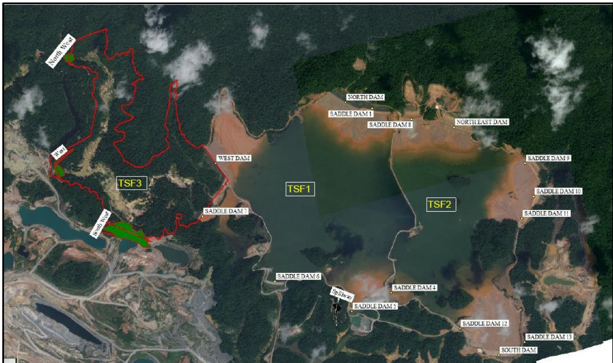
Figure 1: Showing the Current Tailings Storage Facility
